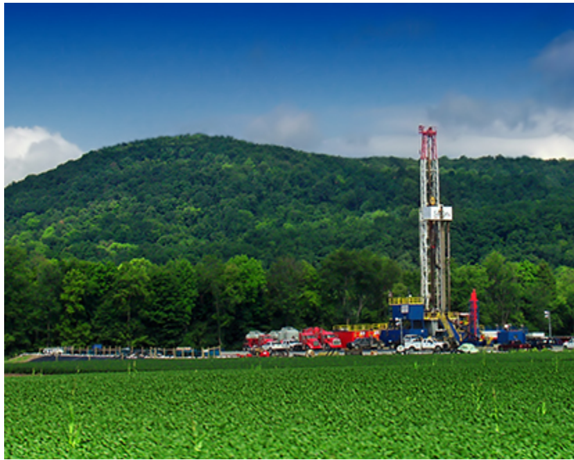
Figure 20.2 This is a Marcellus shale gas-drilling site in Lycoming County, Pennsylvania. (Photo courtesy of Nicholas A. Tonelli/flickr)
